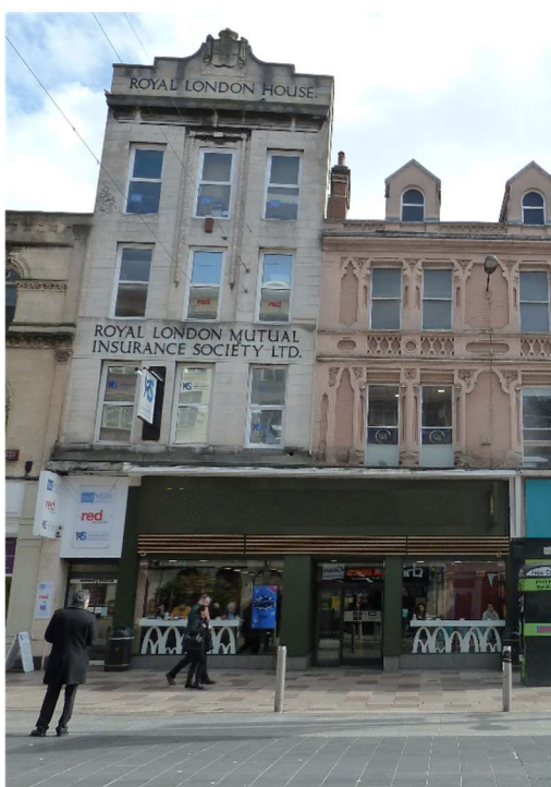
Shopfront does not acknowledge that it spans two historic buildings
